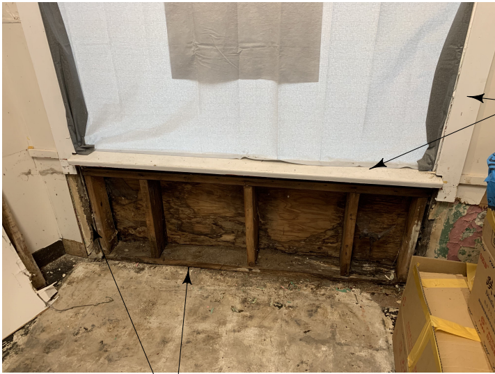
REMOVE FRAMING UNDER WINDOW AND PREPARE MASONRY SUBSTRATE AS NEW ROUGH OPENING
