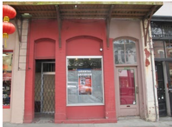
Below: Photos showing existing storefront configuration as viewed from Fisgard Street. Note original door and window openings have been altered at some point in time.
