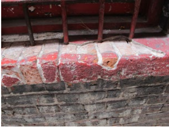
Exposed ground floor sill of 543-545 Fisgard Street facing Fan Tan Alley, showing delamination of parging.
