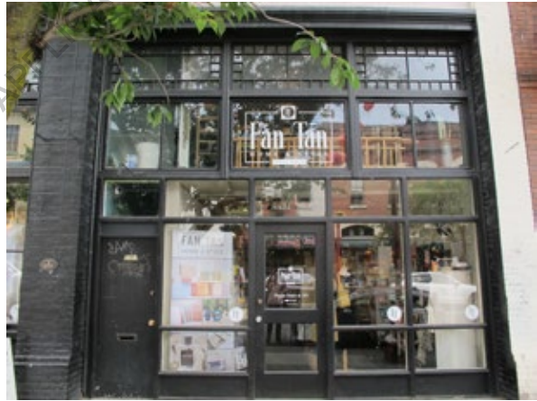
Existing condition of the adjacent original storefront, which is partially shown in the photo above. Note existing replacement door to access upper floor units.
