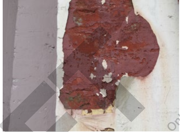
Damaged paint surface of storefront column at 543 Fisgard Street. The brick was originally unpainted. Note peeling down to early paint layers; the earliest application appears to be a red lead hydrophobic coating.
