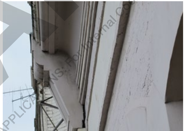
Close-up view of sheet metal cornice, showing detachment from wall surface at east end.
