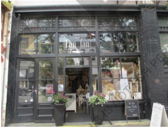
Existing condition of the original storefront shown in the photo above. Note existing replacement storefront door assembly, including sidelights and transom (with decal of address "541").
