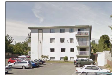
EXISTING BUILDING FROM LEWIS STREET
