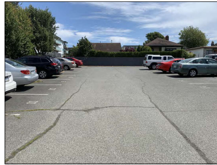
3 A2 VIEW OF EXISTING PARKING LOT
