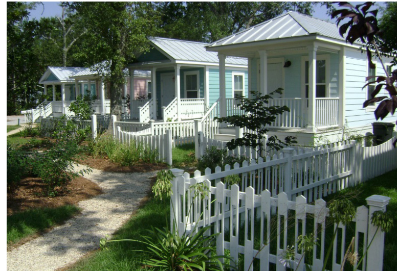
Example cottage cluster style homes on permanent foundations. Cottage Square, Ocean Springs, Mississippi, Bruce Tolar Architect
