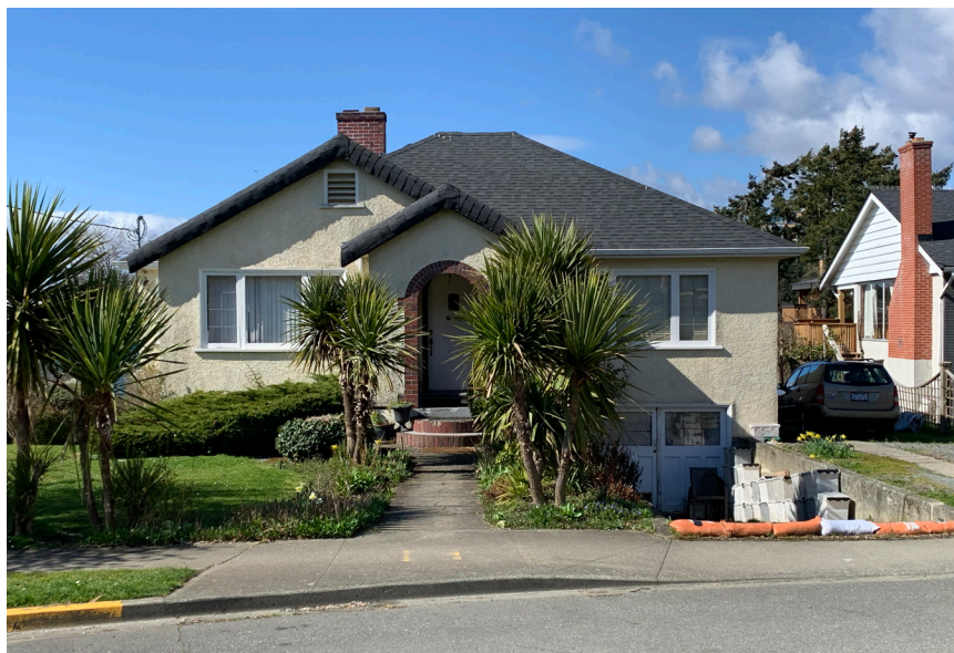
206 Robert Street, c. 1945, Constructed by A. Petek for Mr. George Goy. Rolled eaves and bricks embedded in plaster are references to the English Cottage Style
