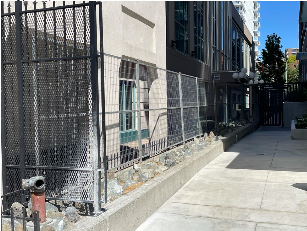
Along property line between 836 and 848 Yates
