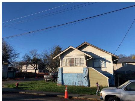
Existing Single Family Dwelling
