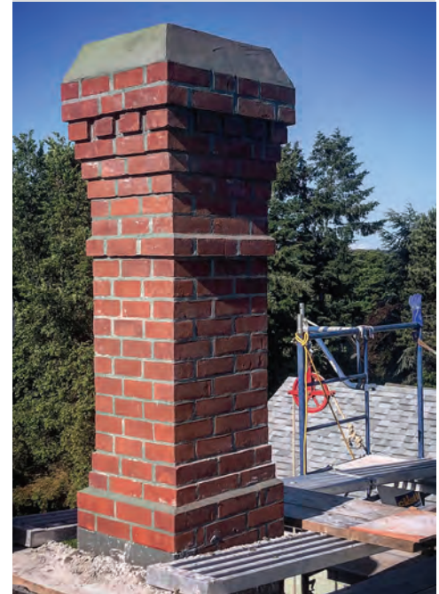
1260 Denman St rebuild chimney
