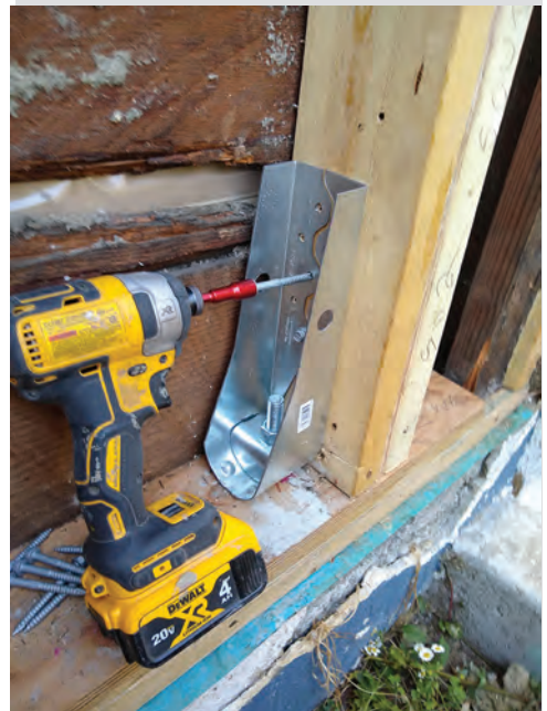
1270 Balmoral Rd seismic upgrades
