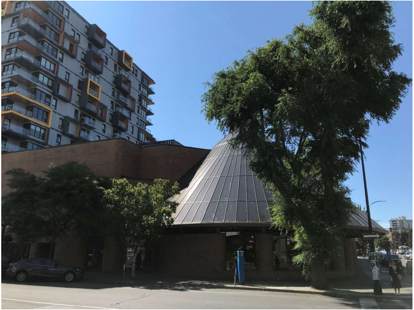
Photograph 7 – Trees 4670-4072 in context with existing building, looking south from Yates St.
