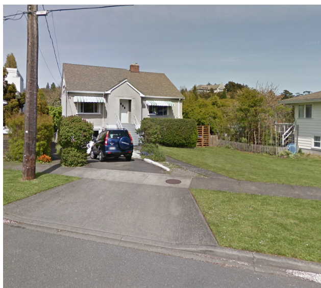
1344 Thurlow Road - Existing Residence
