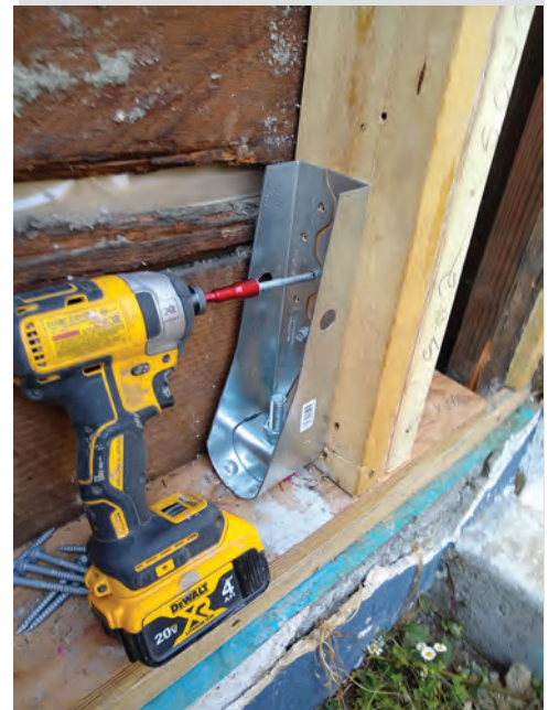
1270 Balmoral Rd seismic upgrades
