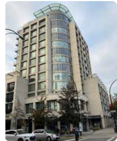
Diagram and photo illustrating a portion of a point tower frontage along a street or open space extending straight down to the ground.
