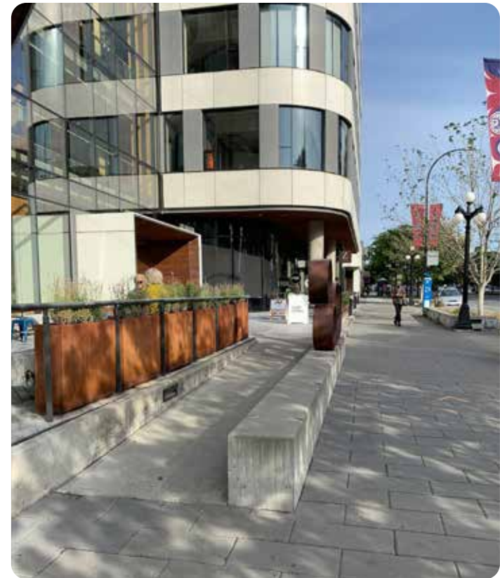
Example of a highly visible access ramp integrated into overall building design.
