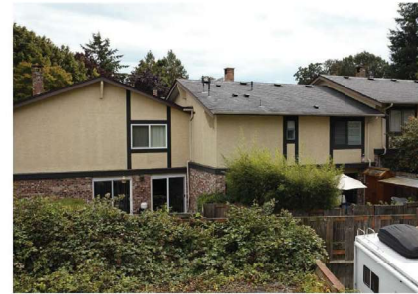
NOTE: 949 PEMBERTON ROAD WINDOW & DOOR LOCATIONS AND SIZES EXTRAPOLATED FROM SITE PHOTOGRAPH ABOVE
