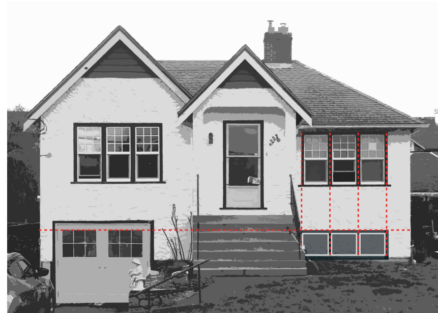
Align new basement windows with upper storey windows and include the same number of vertical divisions.
