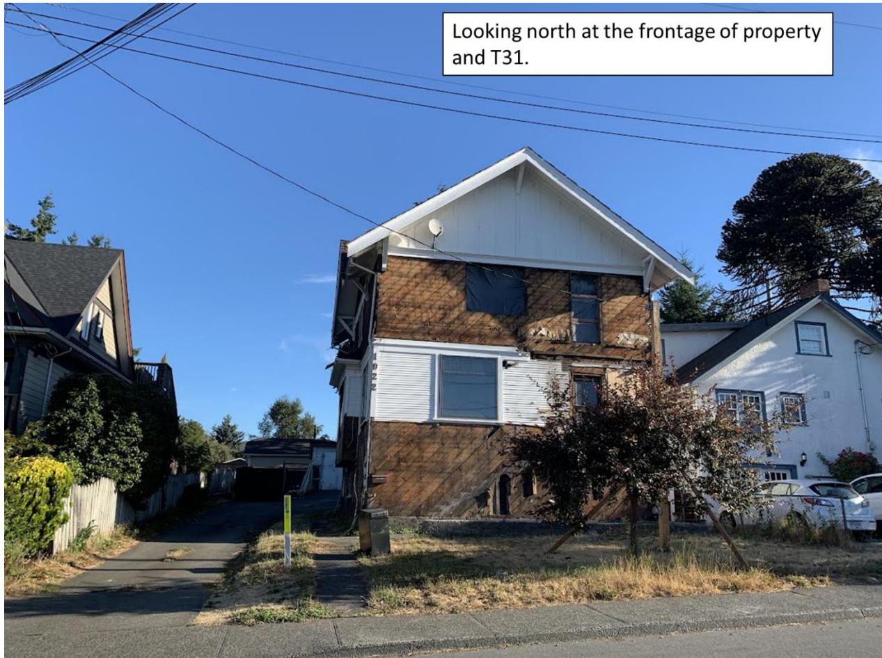
Picture 1 – Looking at the frontage of the property.
