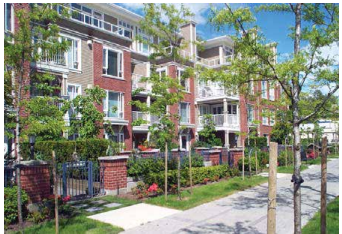
Generous residential building setback along a corridor
