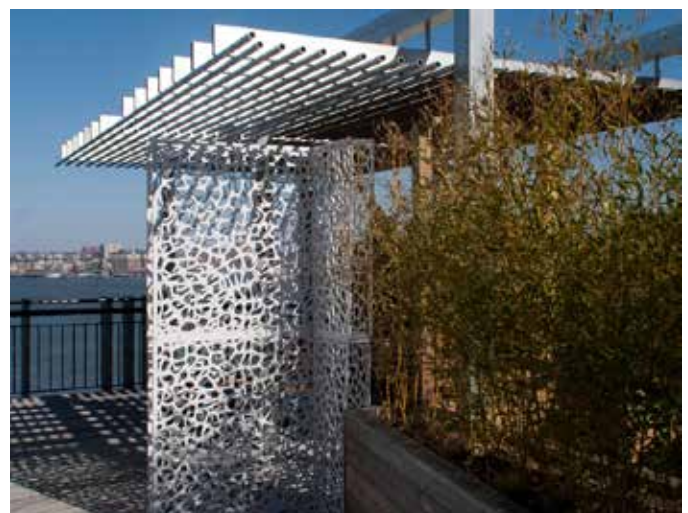
A combination of ornamental grill work and landscaping to screen mechanical equipment
