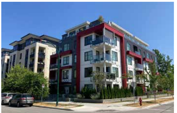
Examples showing different approaches to articulation and variation in facade treatment
