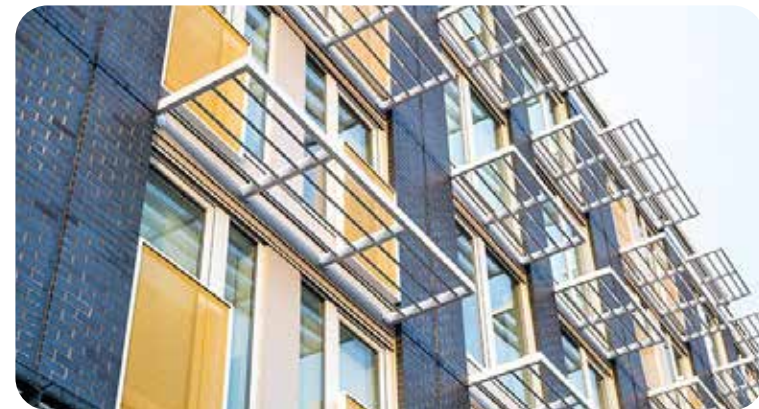
Example of fixed fins and other green building elements as part of the expression and articulation of the building facade.
