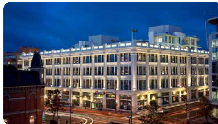
Examples above of lighting as a key element of design of the effect of building facades.
