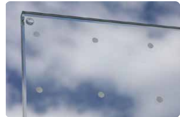
Examples of glass treatments and designs that reduce the likelihood of bird strikes.
