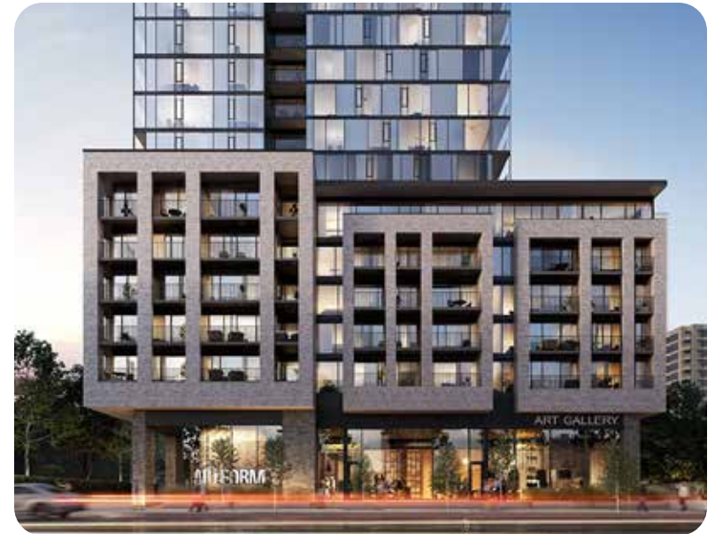
A combination of projecting and recessed balconies can help articulate building mass.
