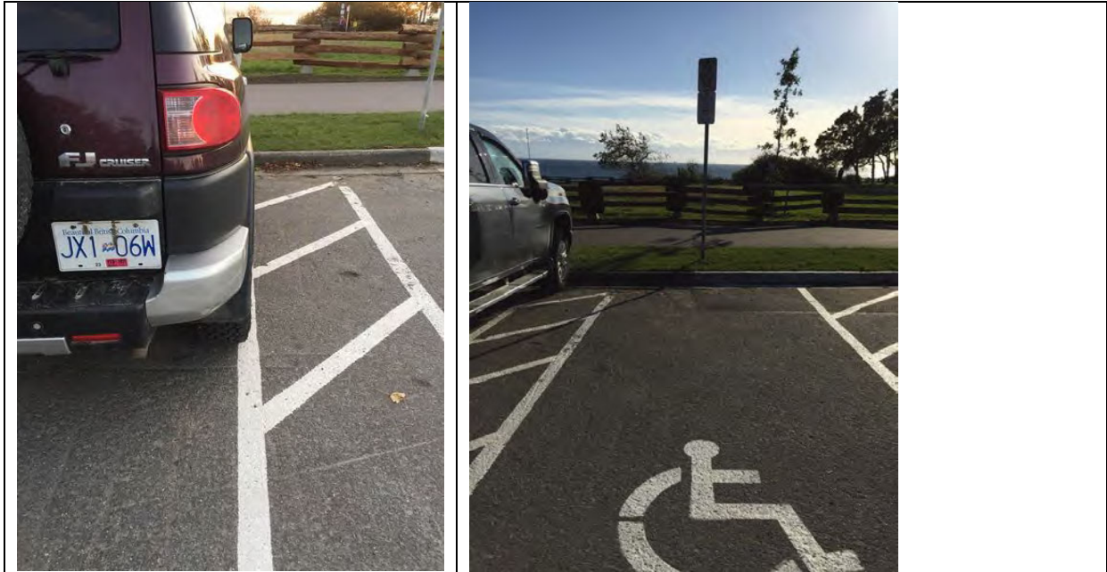
Exhibit 5 – common buffer zone incursions, indicating not sufficient width
