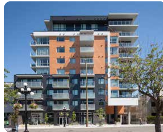
Example of a mid-rise building that articulates its building mass through a combination of vertical and horizontal setbacks and changes in material.
