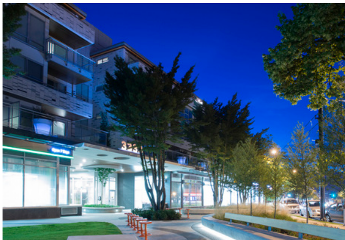
Lighting used to highlight building features and create safety while avoiding over-illumination of the public realm.
