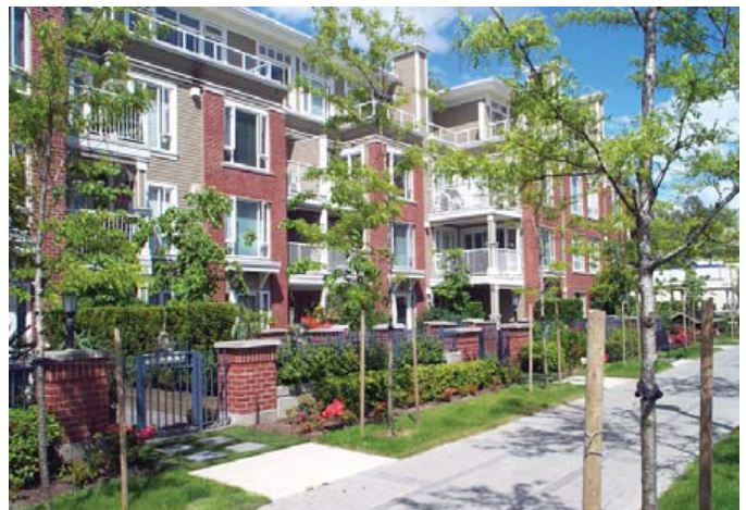
Generous residential building setback along a corridor.
