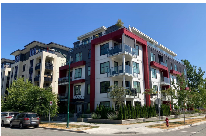
Examples showing different approaches to articulation and variation in facade treatment.
