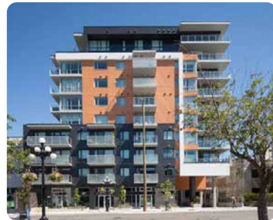
Example of a mid-rise building that articulates its building mass through a combination of vertical and horizontal stepbacks and changes in material.
