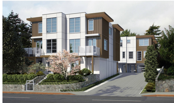
Double row townhouses should be oriented parallel to the street, and provide sufficient building separation and setbacks to ensure liveability for units within the development and on adjacent sites
