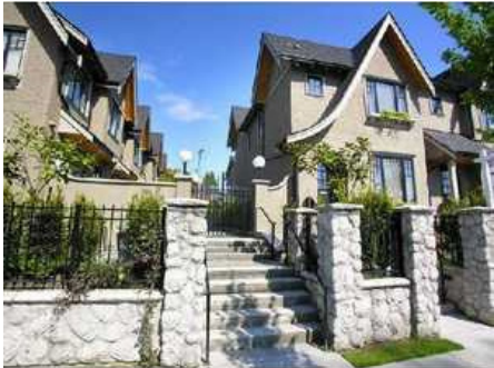
Example showing incorporation of terraces, planters, and stairways to sensitively transition the grade.
