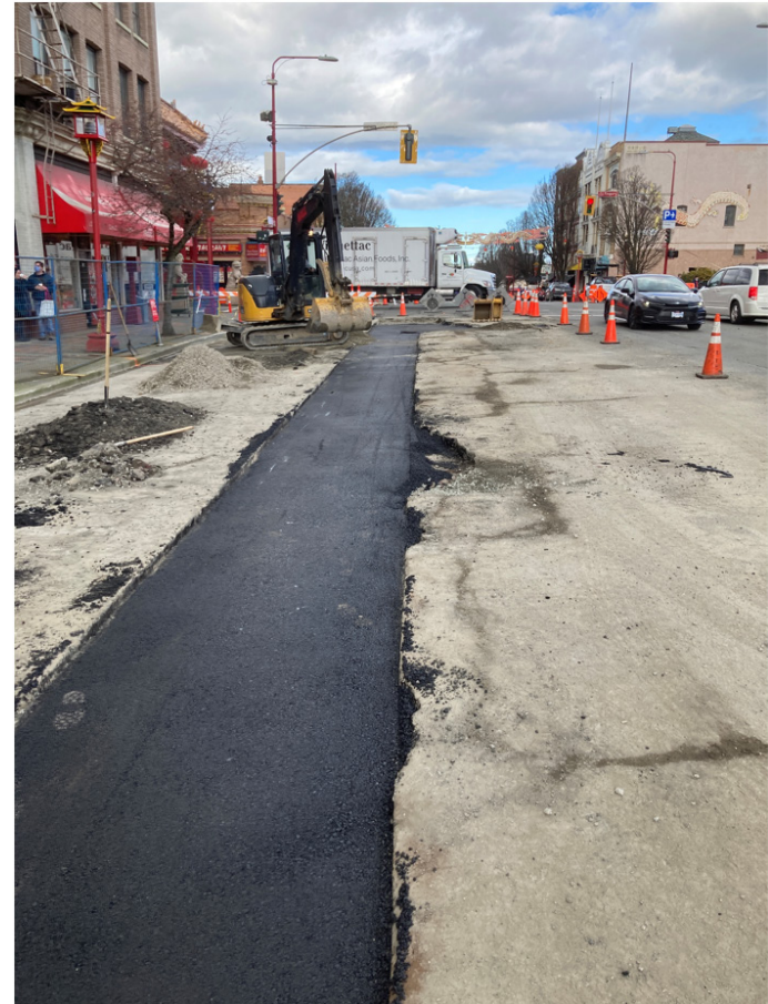
A photo taken during the now completed construction of water main replacement and BMP network North of Pandora Ave.
