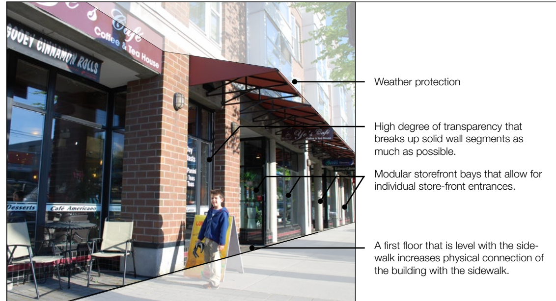
Ground Floor Commercial Components
