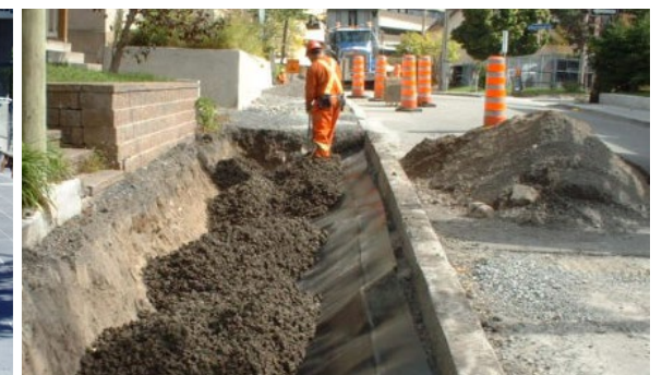
Structural soil installation
