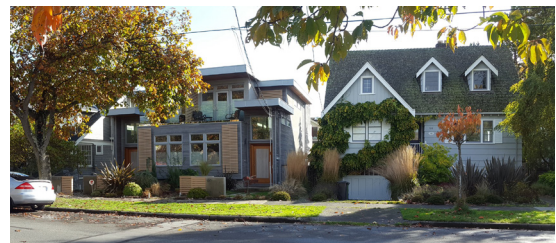
Compatible forms with contrasting architectural styles add diversity, character and visual interest along a street.
