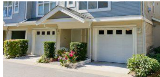
Example showing incorporation of landscaping to soften an interior drive aisle and emphasize entries
