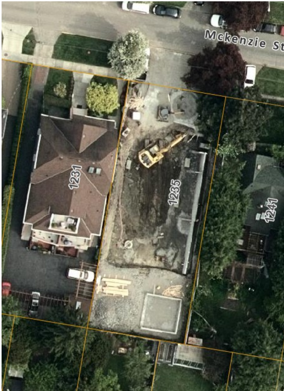
Imagery from 2015 demonstrating the removal of all green space and trees to facilitate construction.
