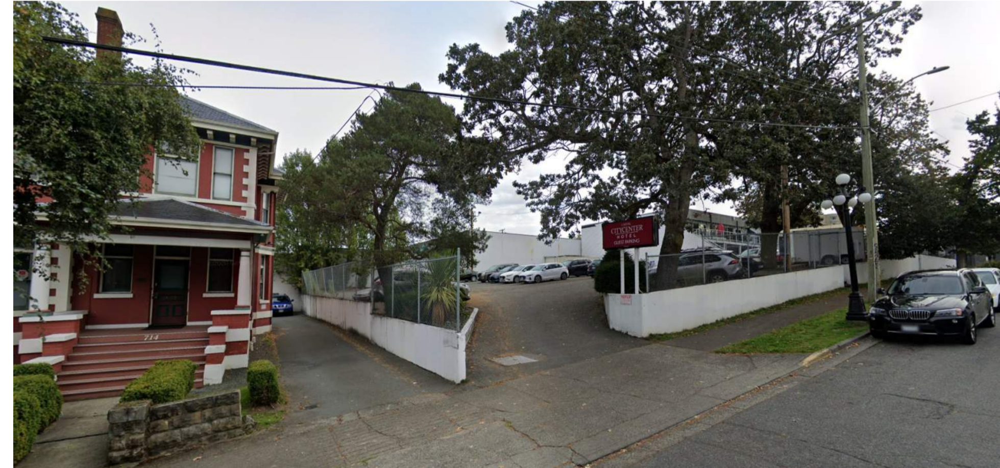
3 Looking North-East DP0.1
