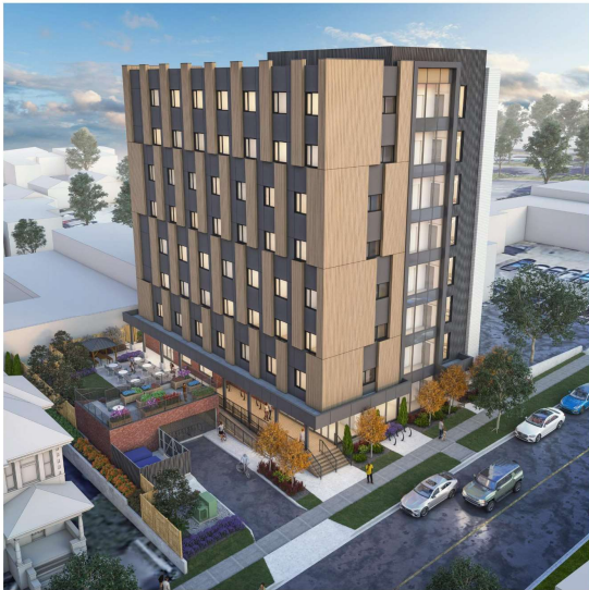
AERIAL VIEW LOOKING NORTH-EAST
