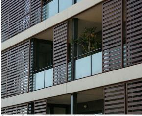
Sun shading screens integrated into façade
