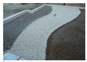
Roof treatment using light and reflective colours to minimize urban heat island effect
