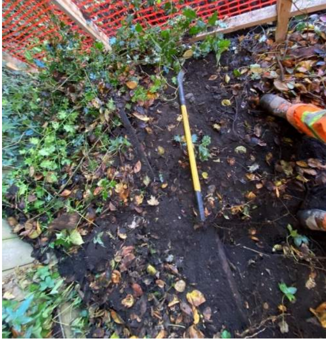
Photograph 3: 10cm root encountered at 1m from Southeast property corner (approximately 5cm below surveyed grade).
