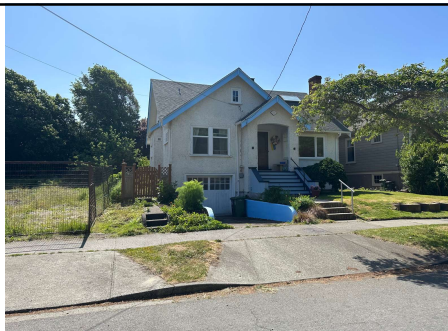
South-west side of site
