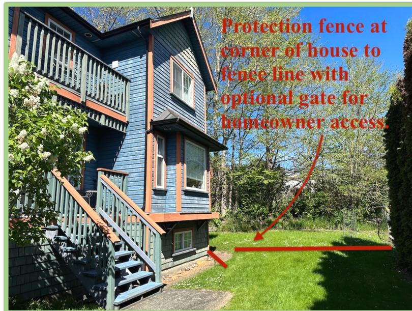
Although this fence does not fully capture the root zones of the stand of trees, the protection buffer will stop material storage or unintentional vehicle and machinery impacts to the areas closest to these trees. Fence removal for construction access to this area will require arborist supervision or direction. *See attached basic site plan.*
