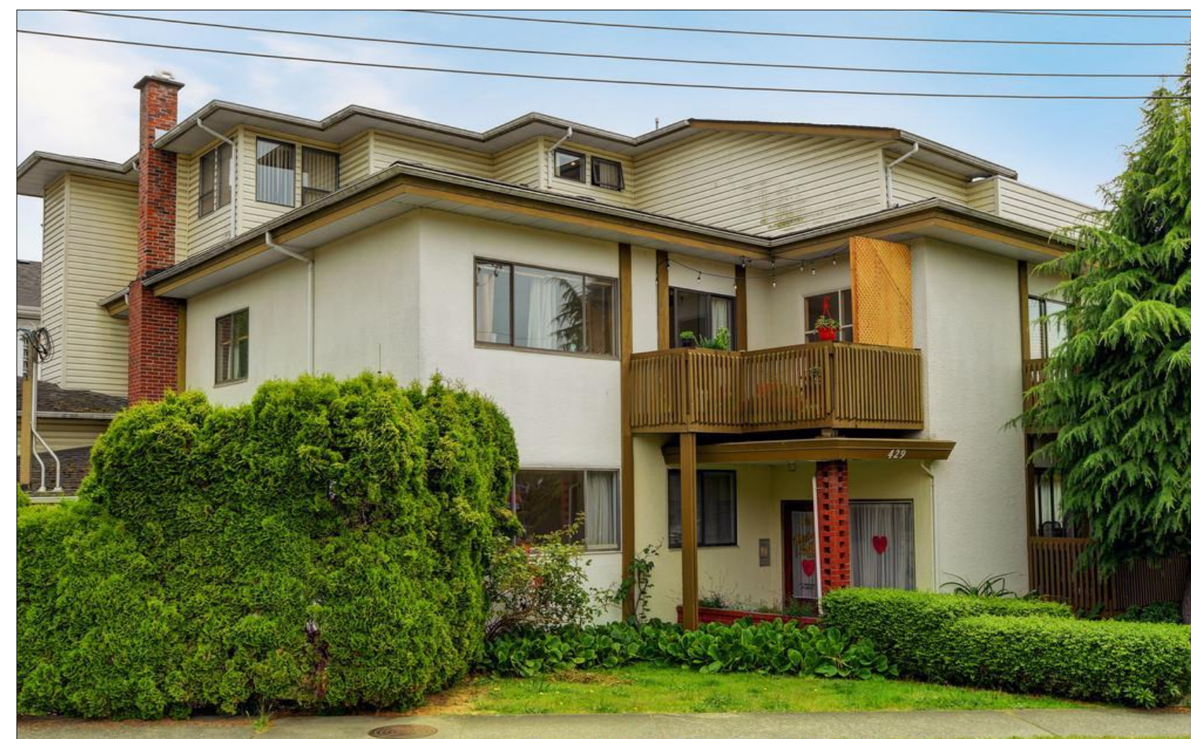
EXISTING BUILDING VIEW FROM VANCOUVER STREET
