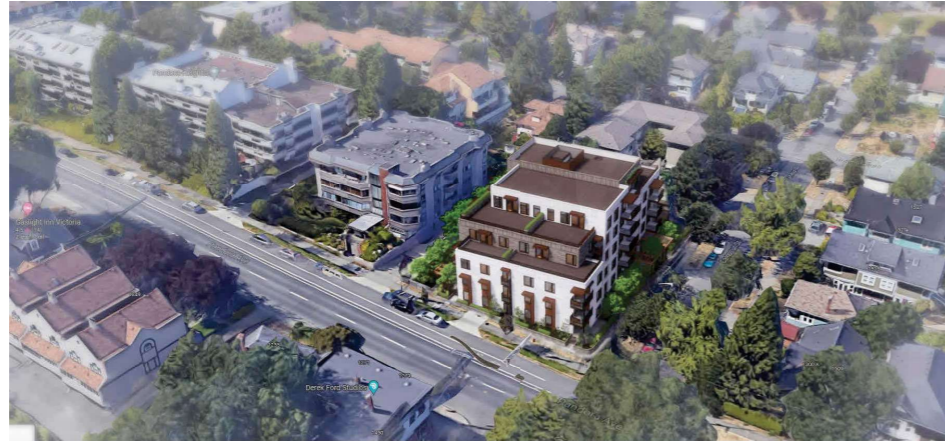
View from Pandora and Camosun looking Northwest
