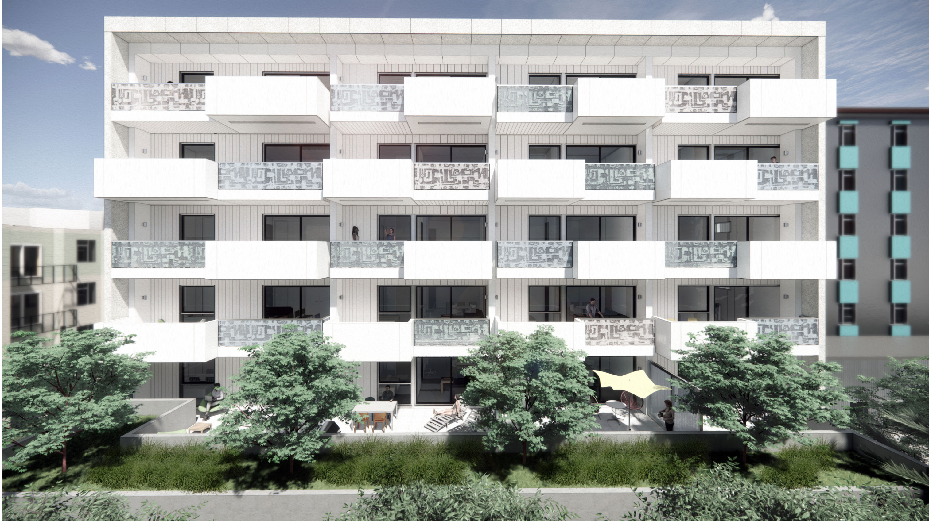
VIEW OF SOUTH FACADE
