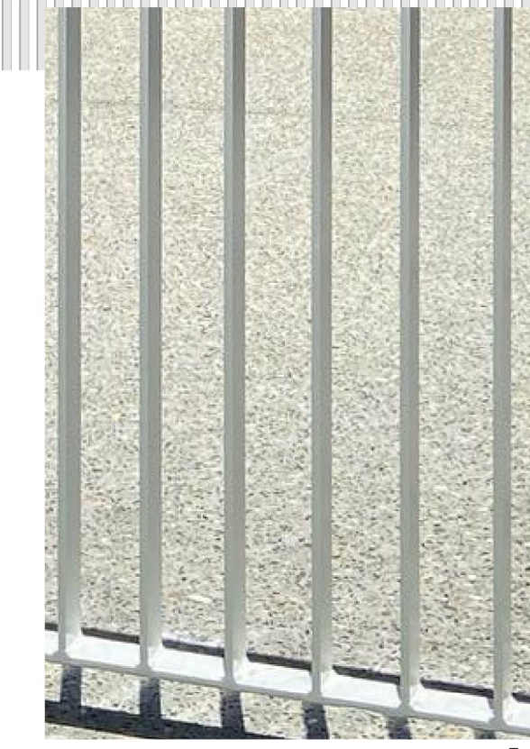
7. METAL PICKET GUARDRAIL [WHITE]
