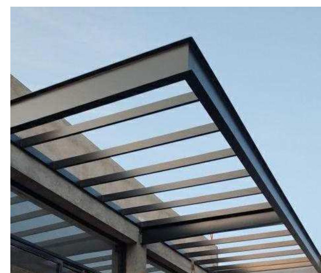
BLACK PAINTED STEEL CANOPY W/ LAMINATED GLAZING
