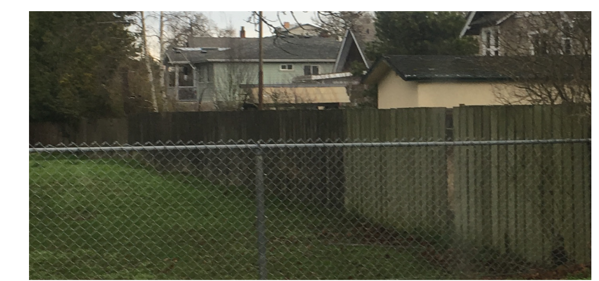
Existing fence panels. New fence to match existing fence.
