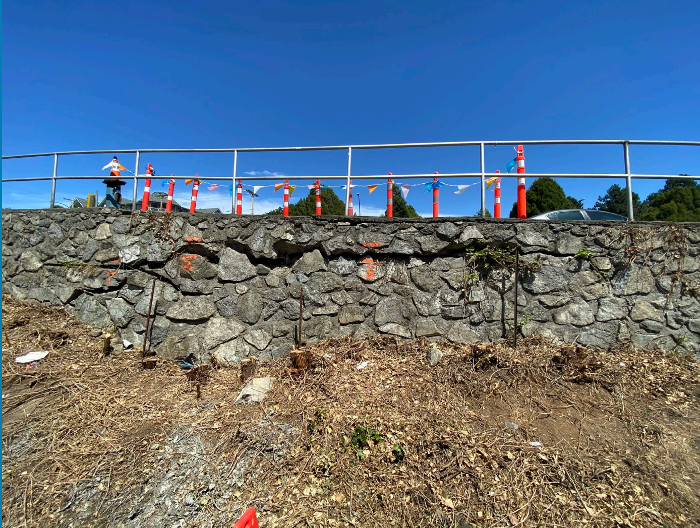
Examples of wall in Failed Condition
