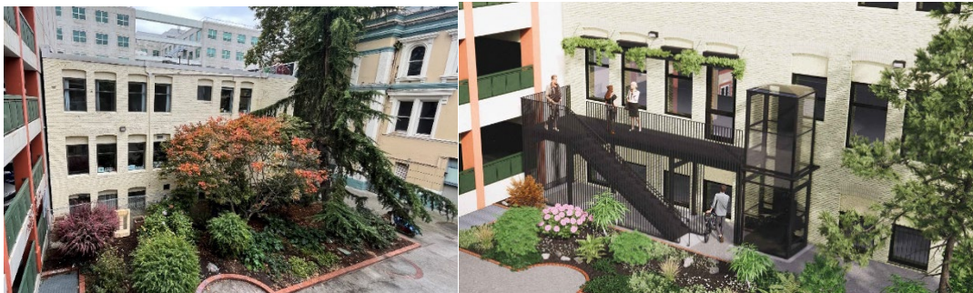
Images left to right: Image of current condition of rear of 1218 Langley facing Chancery Square; Design proposal of stair, lift, shutters and trellis at top of windows to hide shutters.
