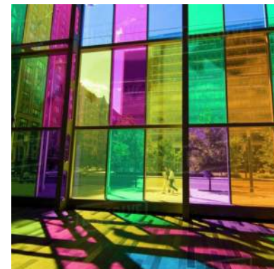
Window Wall System w/ Low E Insulated Glass & LED Coloured Backlit Feature Wall
