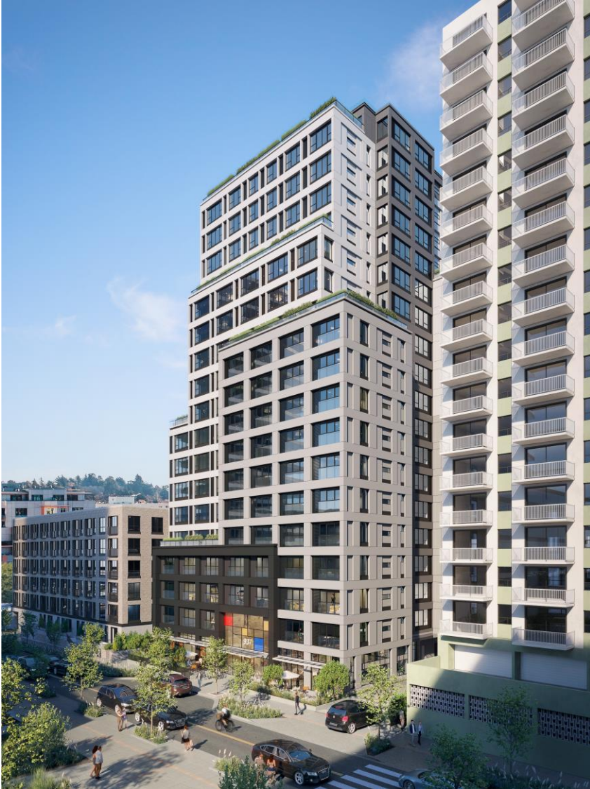
Overall project view from North / West.
