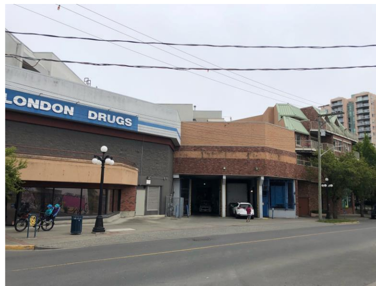
View of North neighbour (Harris Green Commercial Complex)
