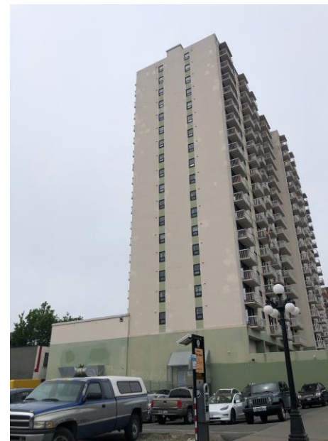
View of West neighbour (View Towers)
