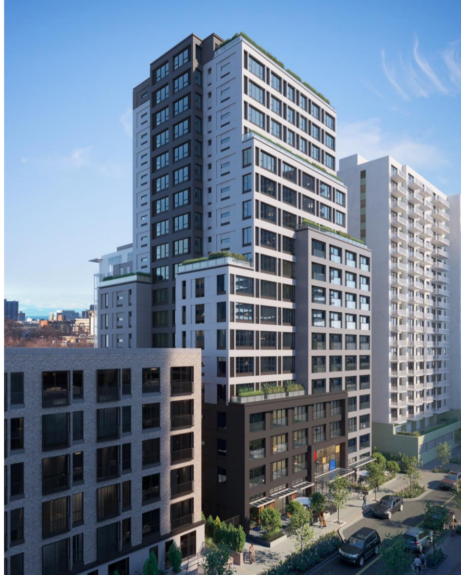
Overall project view from North / East.
