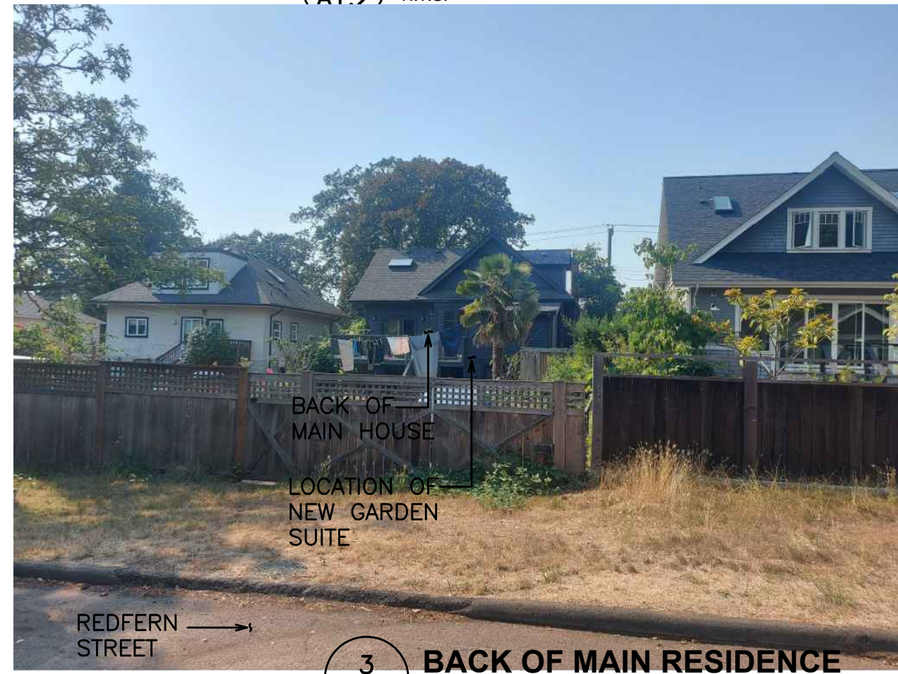
3 BACK OF MAIN RESIDENCE A1.2 N.T.S.
