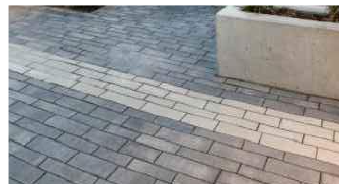
DRIVEWAY: PERMEABLE PAVERS
