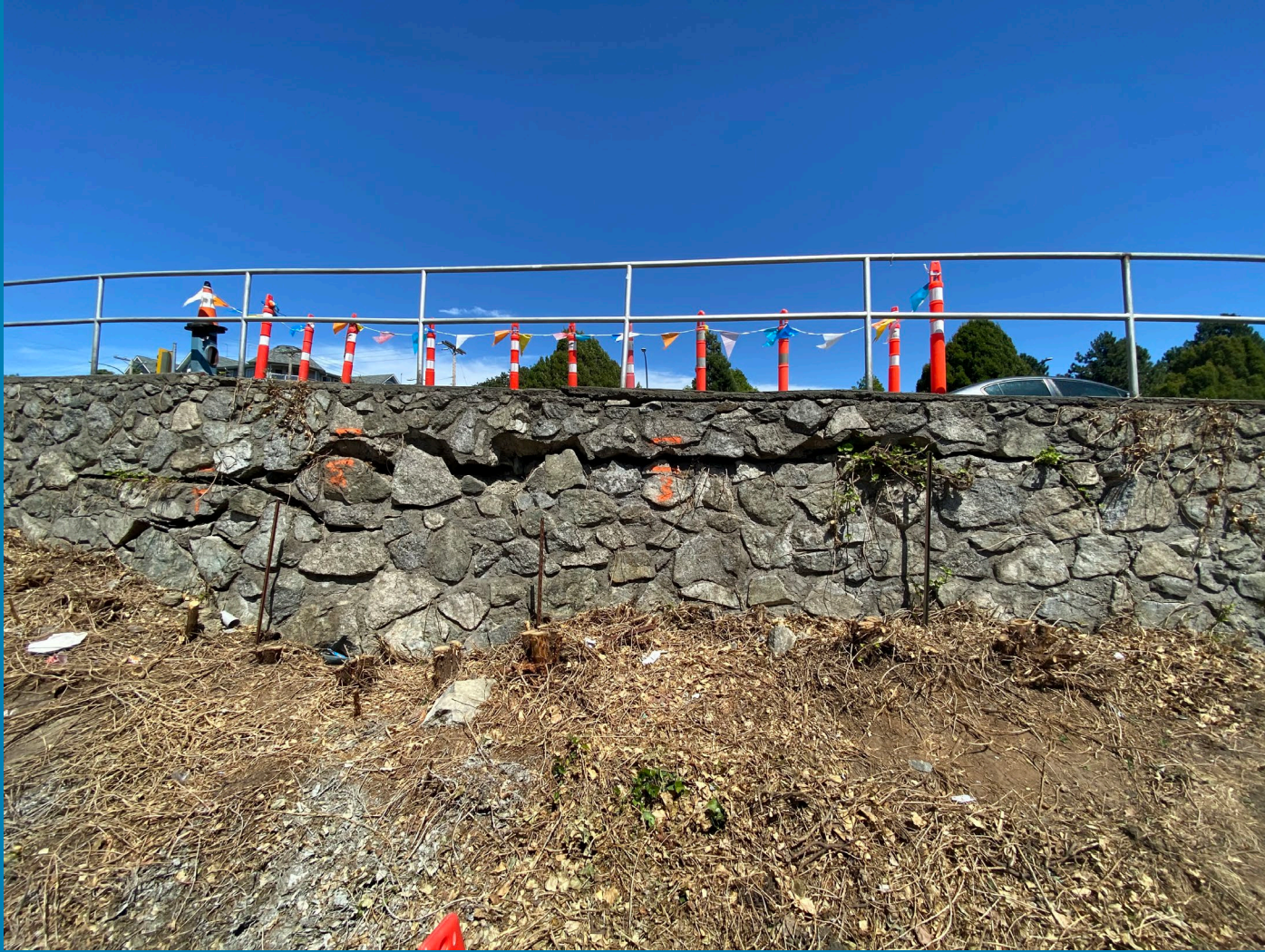
Examples of wall in Failed Condition
