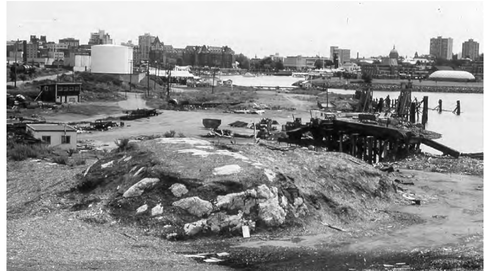
Site looking east, 1983
