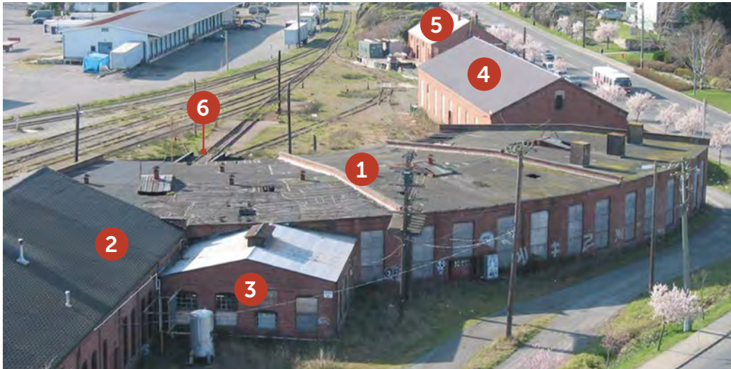
Roundhouse, view from east, with Backshop and Boiler House Photo: City of Victoria (2003)
