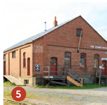
Stores building, view from east (Focus Equities)
