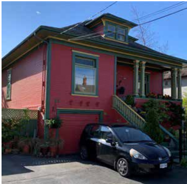
35 Lewis Street, built 1907.
