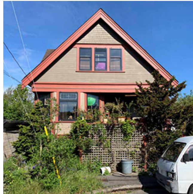
50 Lewis Street, built 1912.
