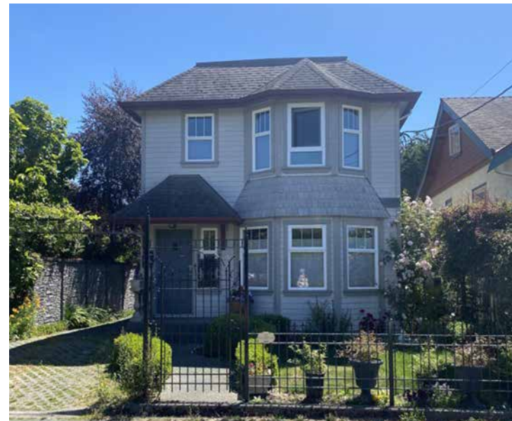
27 Lewis Street was built in the 1990s and fits well within the street. Its form, scale and massing are all sympathetic to the context, and the details and features such as the angled bay and covered front entry are modern interpretations of common features of the historic homes on the street.
