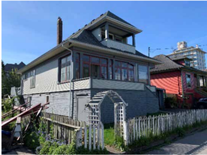
39 Lewis Street, built 1908.
