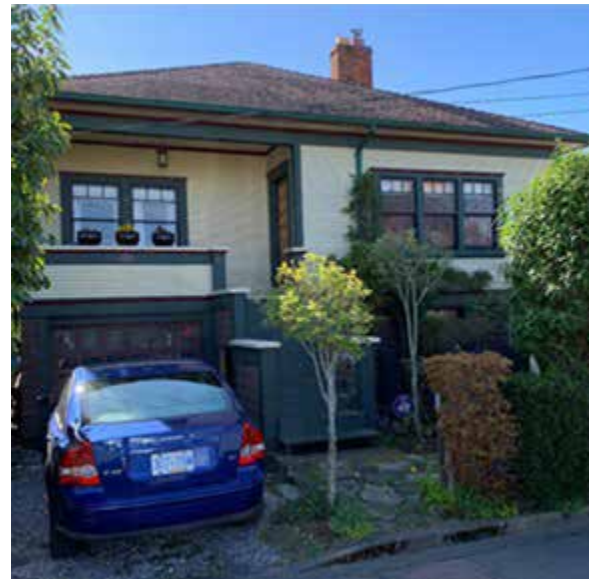
53 Lewis Street, built 1929.
