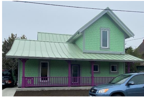
44 Lewis, under construction
