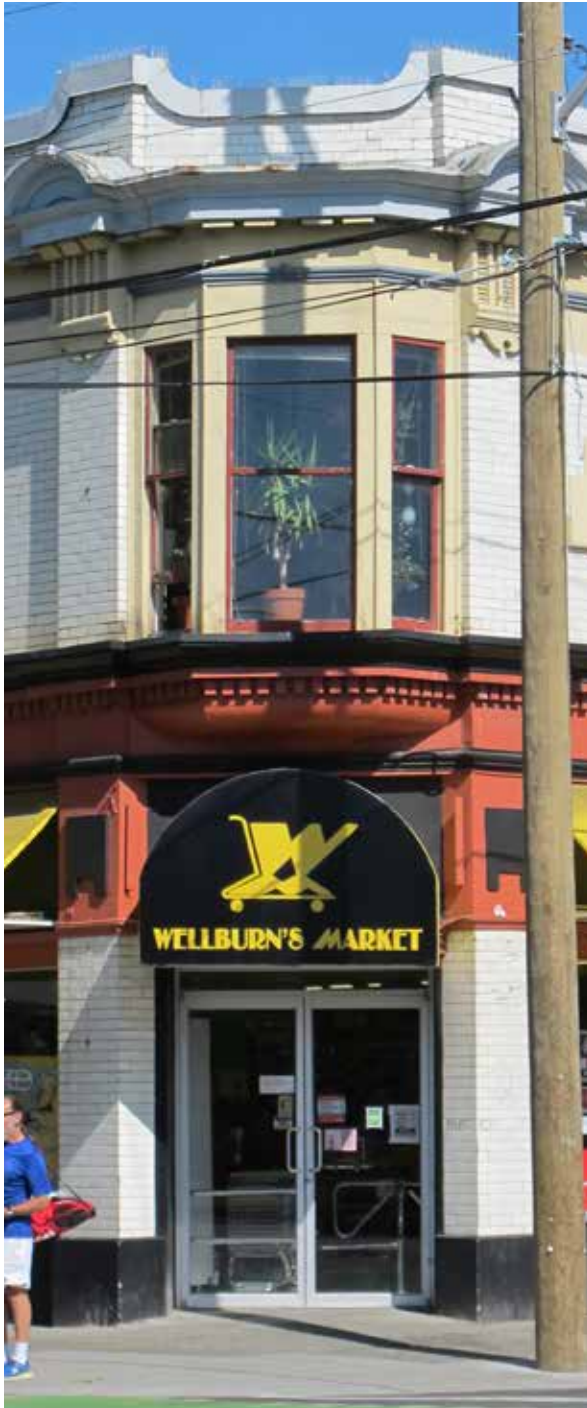
Above: Chamfered entry on ground floor with double doors and transom (hidden by awning). Historic assembly has been replaced with aluminum assembly, including transom.
