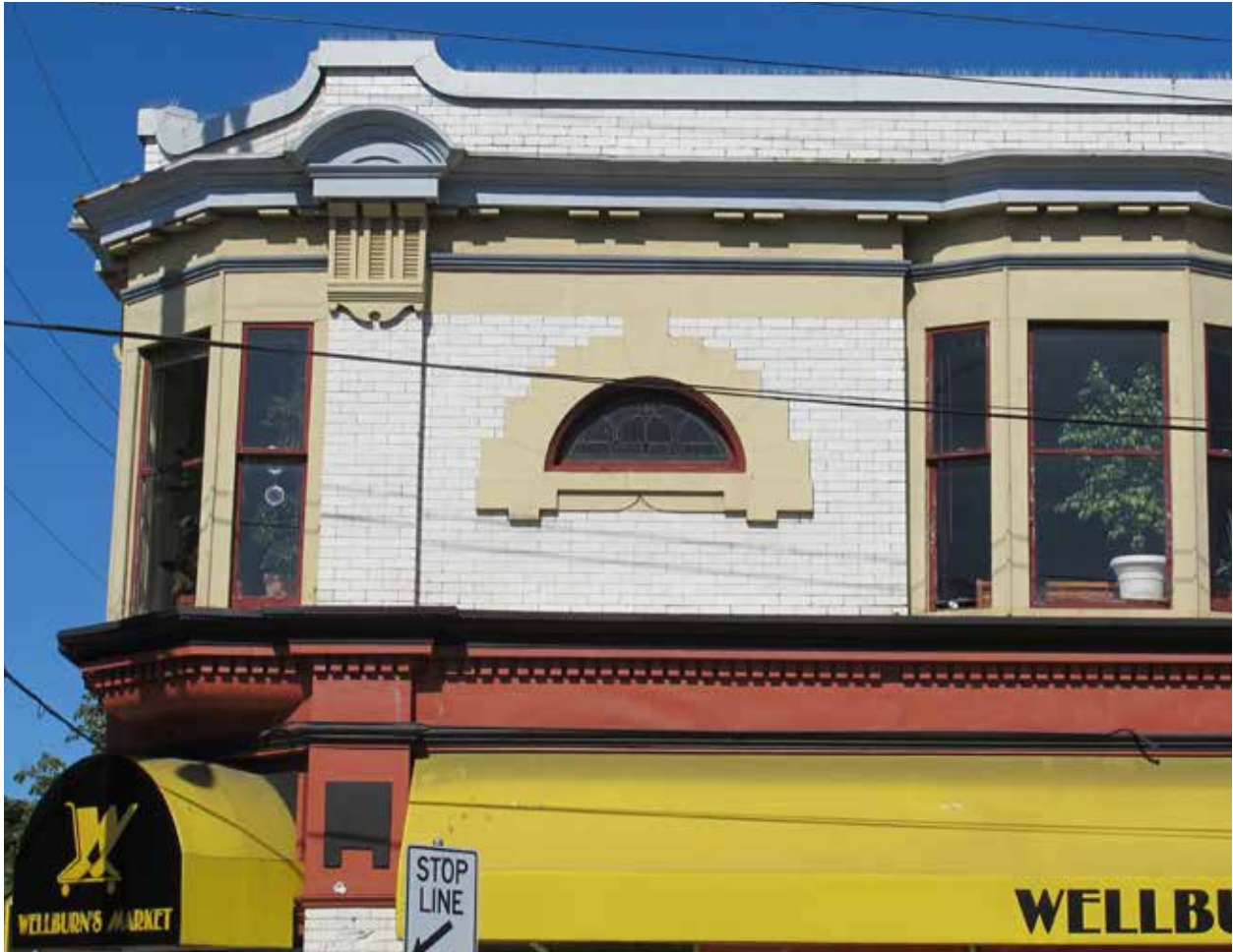
Above: Architectural metalwork of the storefront cornice, brick piers, oriole windows, roof level cornice and parapet cap.
