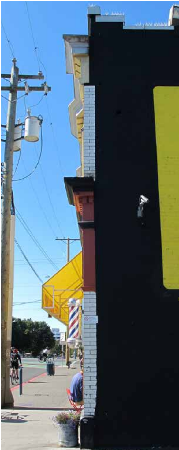
Above: Profile of storefront and roof level cornices that are present on Pandora Avenue and Cook Street façades.
