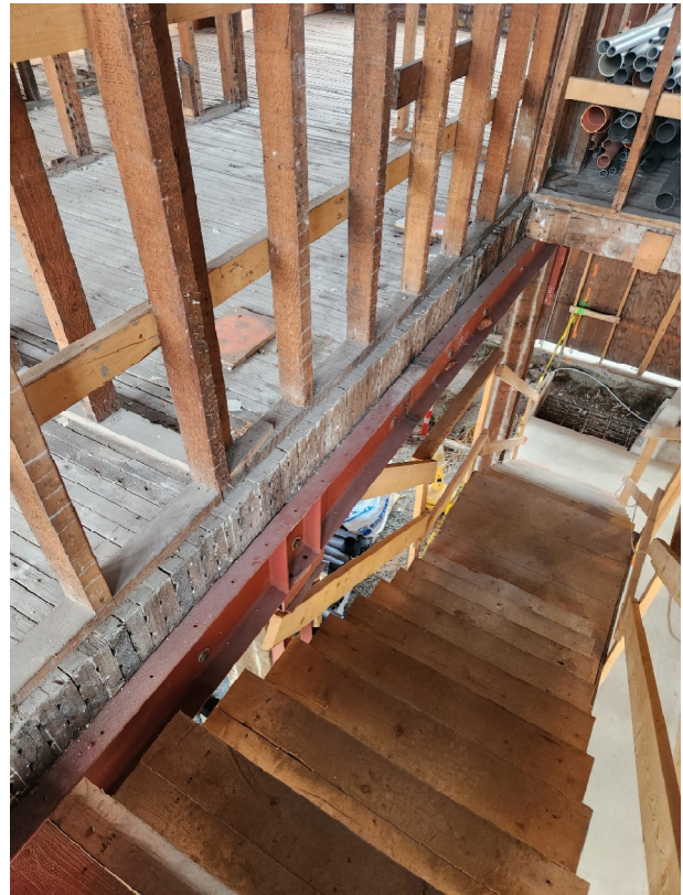
Figure 6 – Stair Opening Cut through 2x8 Floor
