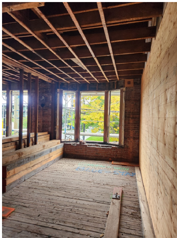
Figure 7 – Typical Second Storey and Roof Framing
