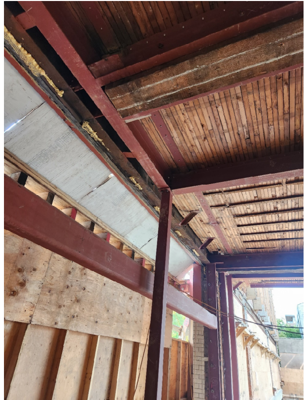
Figure 4 – Underside of Second Storey
